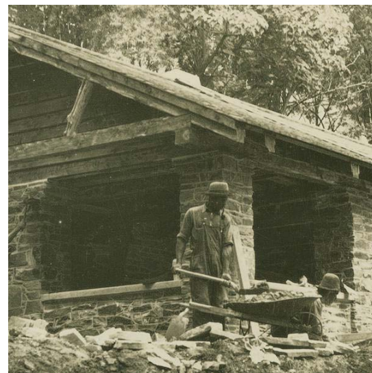
WPA Project Number 319 - Workers constructing stone masonry shelter at the State Teachers College (now Towson University) ca. 1935. Maryland Department Photograph Collection, Enoch Pratt Free Library. [mdpa 113]
